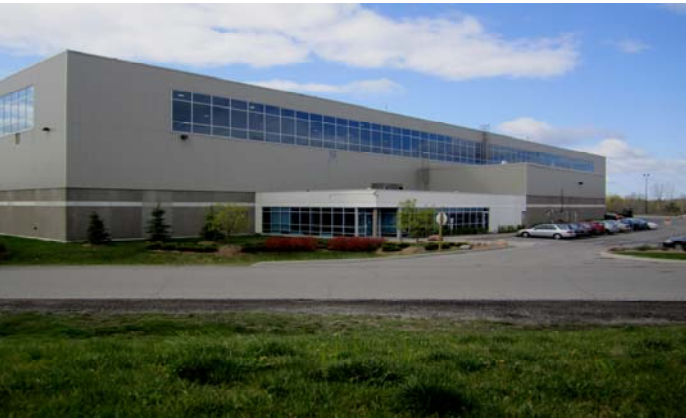
Material Recovery Facility, Whitby
